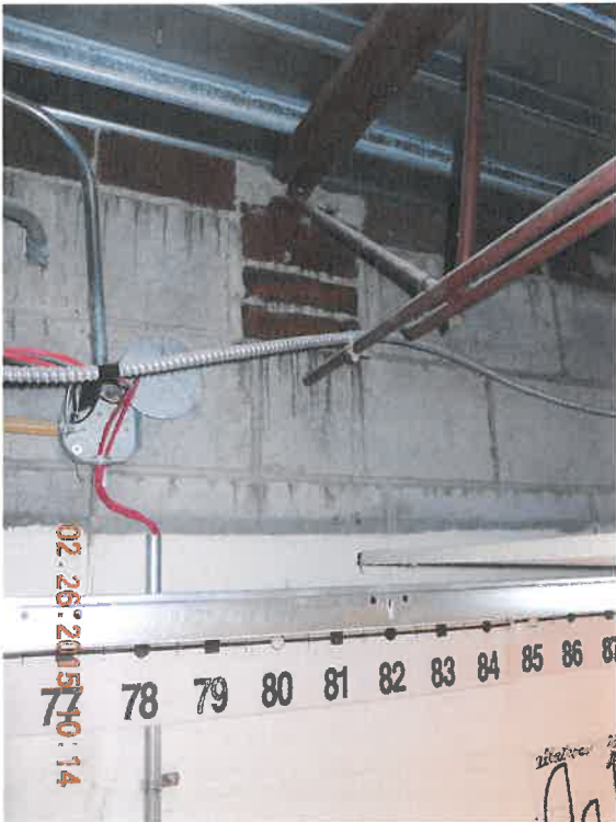
Room 7 - no structural damage observed
