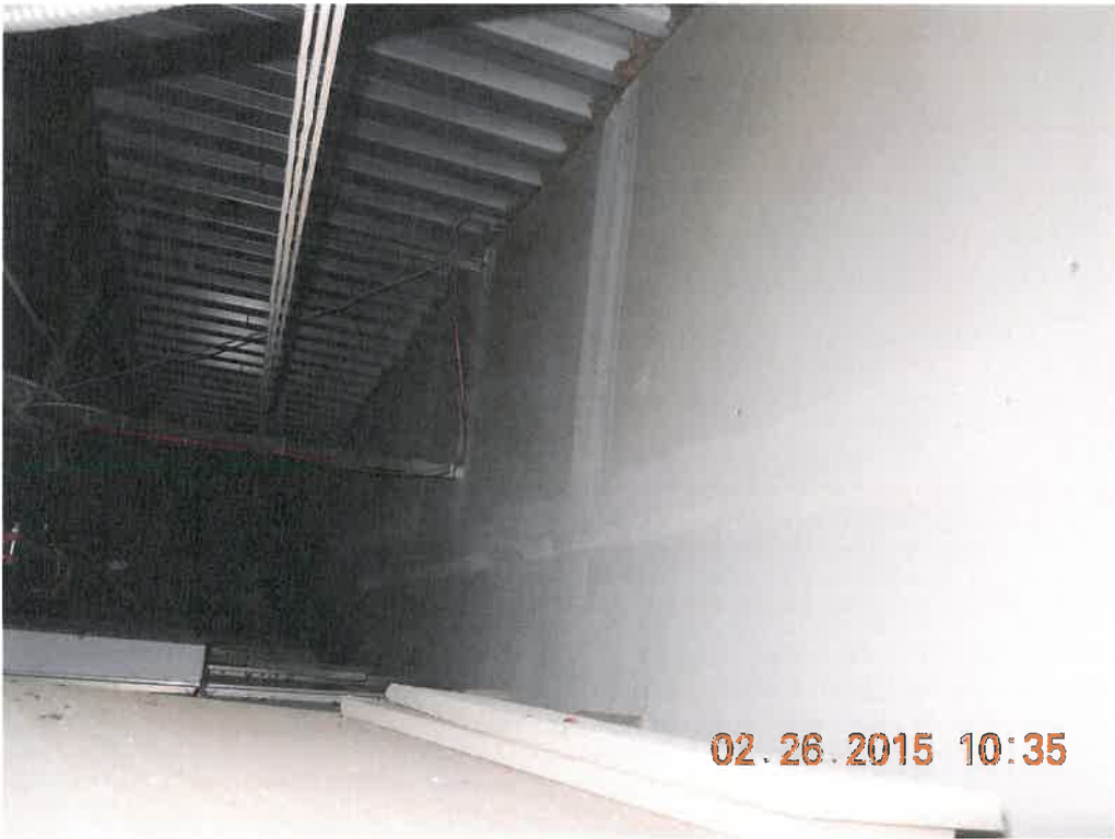
No signs of structural damage
